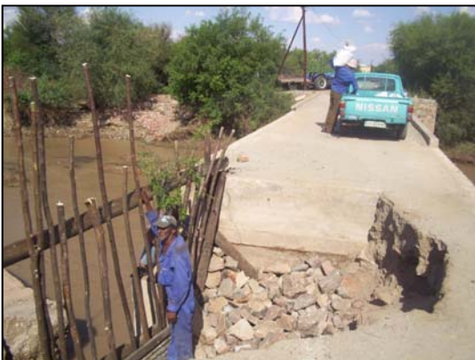
Emergency bridge repairs
