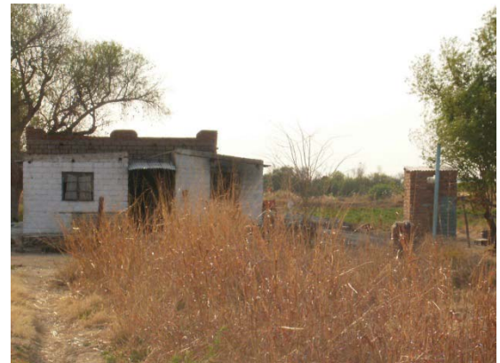
Figure 20: A dwelling on South Island which still has a hole in the roof caused by hail in 2002. Water has to be collected from an open channel nearby.
